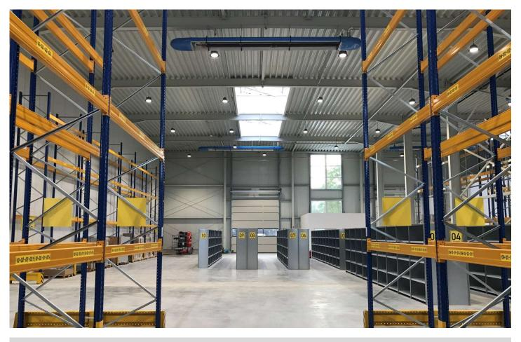
In the newly built 8m high hall, a wide variety of industrial materials such as large wire containers are stored in the high-bay warehouse area. In the front area, medical technology products are stored on lower shelves. The task was to combine the horizontal and vertical LED lighting of the warehouses with optimum illumination of the shipping area.
