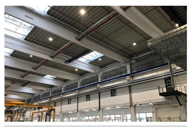
The new production hall is designed for 3-shift operation. Due to different work tasks and visual performance in the room, special demands were placed on the new BuR Lighting LED lighting. The influence of daylight had to be considered. The light colour was set at 4,000 Kelvin.
