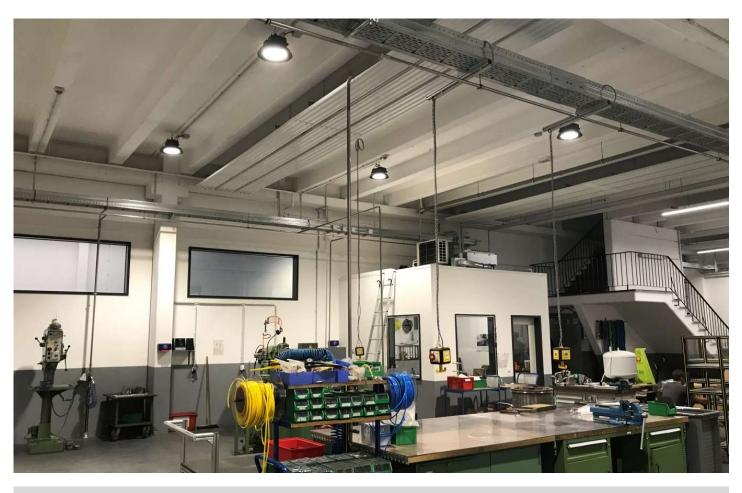
The fixture construction for very special, production-specific fixtures and tools should be rebuilt. The machines had to be relocated. The lighting requirements were no longer met. Illuminance in the working plane was too low for the visual tasks required. The lighting costs were too high.
