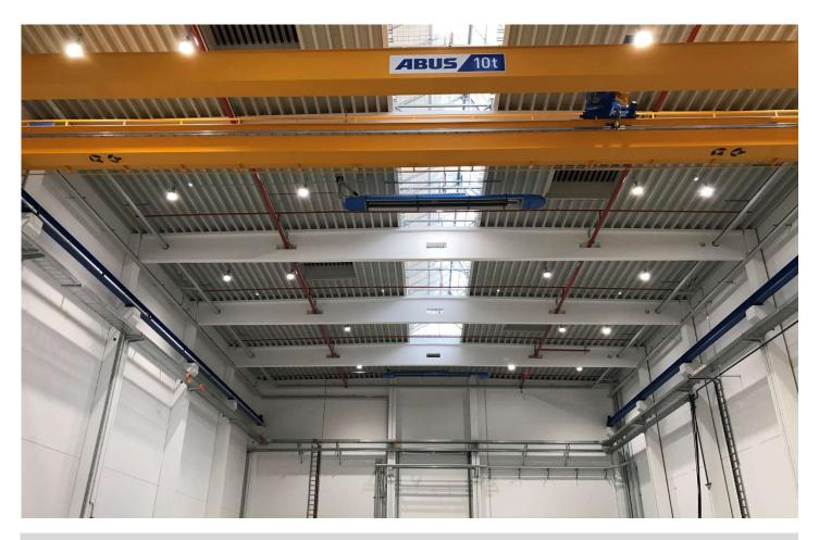
The new hall for surface plating is designed for 3-shift operation. Due to different tasks and visual performances in the room, special demands were placed on the new BuR Lighting LED illumination. The light color was set at 4,000 Kelvin. The energyefficient new illumination should result in an optimum illumination of the surfaces.
