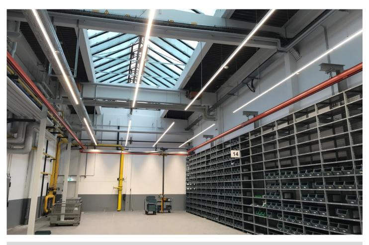
The small parts warehouse for tool sets was newly furnished and was no longer adequately illuminated due to the new arrangement of shelves and storage areas. The conventional illumination did not consider the illumination of the vertical surfaces.
