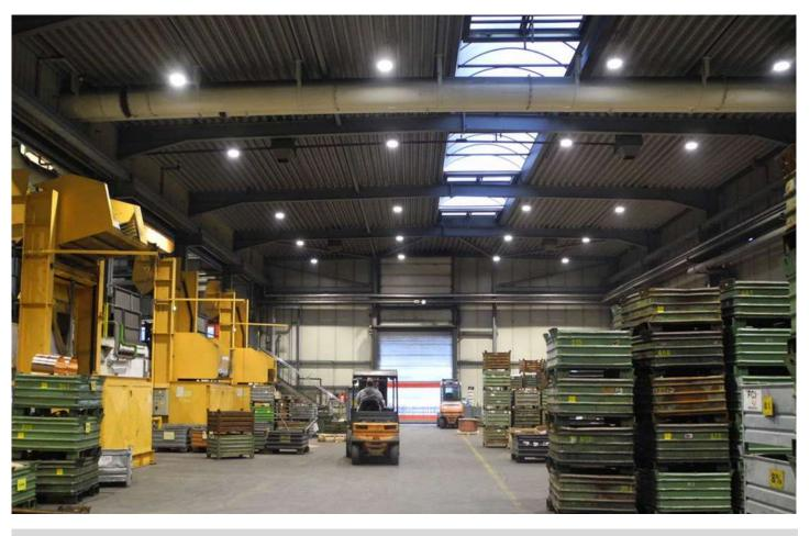
In the stocking area high quality and precious metal parts are stored in large metal boxes. The technical illumination requirements, in particular for the quality of colour rendering, were no longer met. The illuminance in the working plane level was too low. The maintenance costs were negatively affected by frequent lamp changes. The existing 400W high pressure mercury vapour lamps were in continuous operation and no longer up to date.
